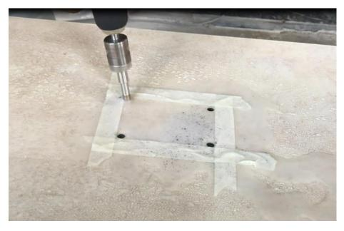
Complete the slot by cutting the slab using a portable circular saw so to connect the holes that have been drilled. Even in this case, keep the area where the cut is being performed constantly wet. Once that all the sides of the notch have been cut, it will be possible to remove the area of Vetrite that has been isolated, completing this way the slot or notch.
