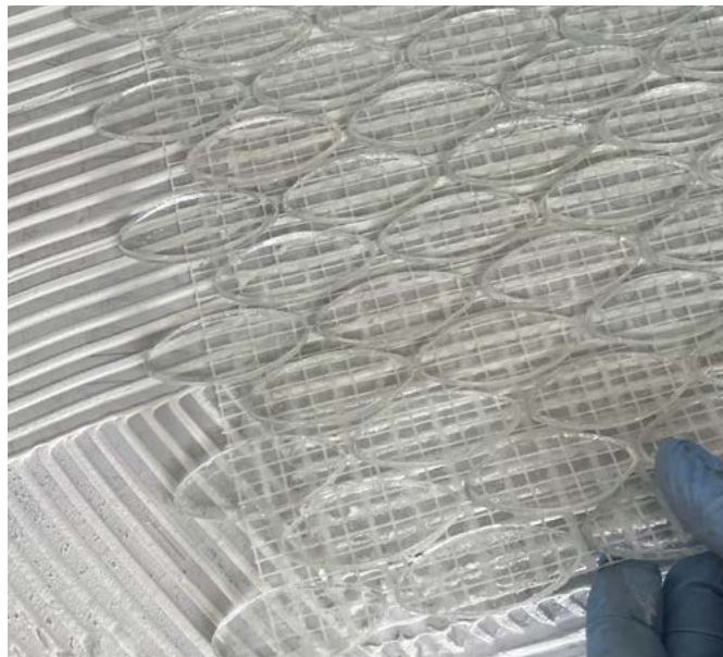
5 Start installing clear glass mosaic
