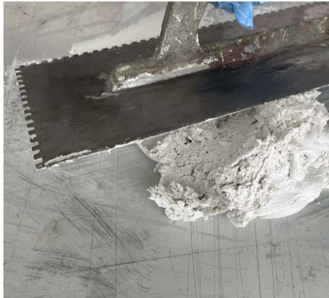
2 Start laying the white adhesive by trowel teeth
